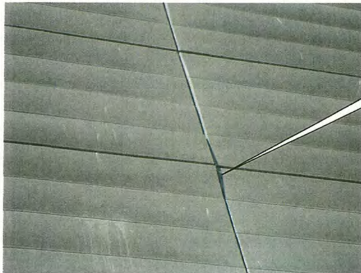
Photo 4 – Several Zinc panel dislocating from their support structure
